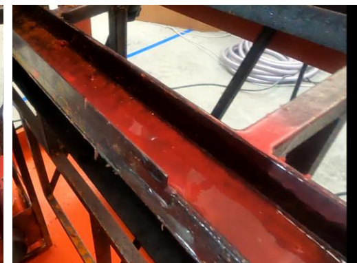
View after spraying
