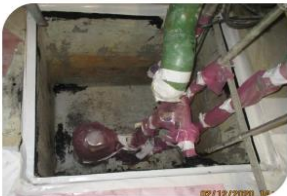
Repair of the tightness of a sump
