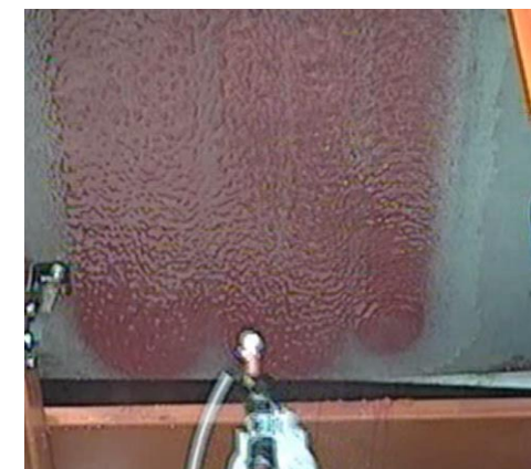
Coating in progress – first layer
