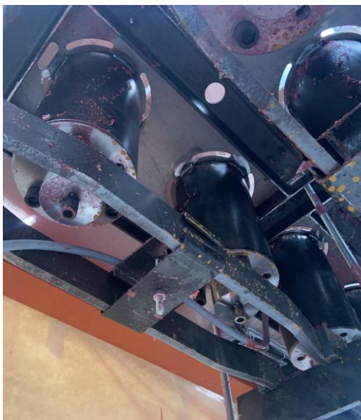
Pictures illustrate the robotic arm was able to spray coating between the CRD-H and that all the surfaces are correctly coated with a 2 mm layer.
