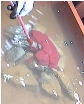
Injection on concrete pieces
