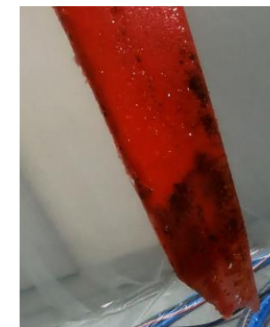
Coating after it has been peeled
