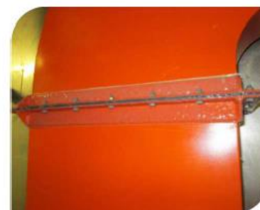
Repair of the tightness of a ventilation duct
